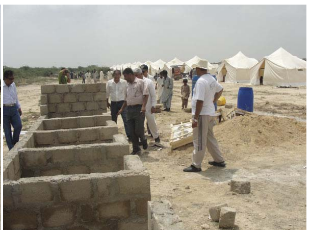
Toilets under construction - so far 12 are already built
