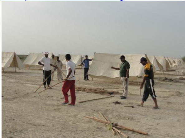
Tents being installed by our workers
